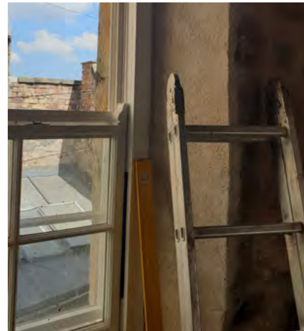
History preserved Traditional materials including lime plaster were used in this retrofit
