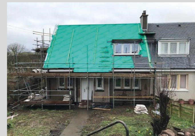
During: grounds cleared and works
