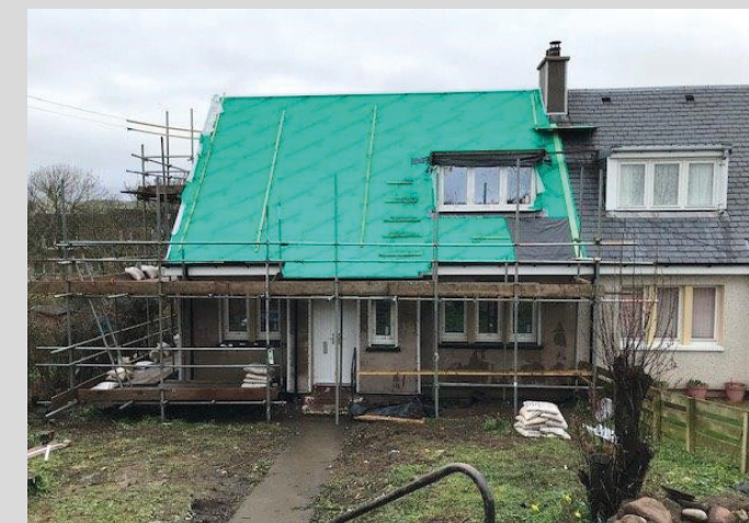
During: grounds cleared and works
