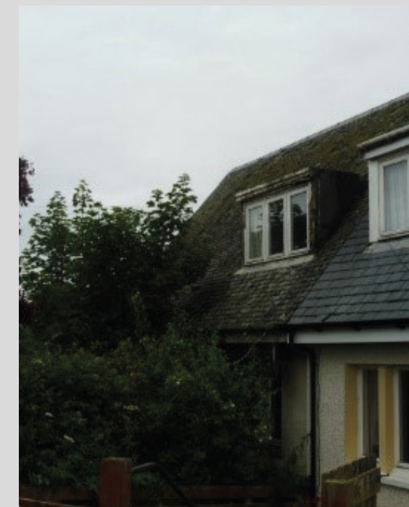
Before: property inaccessible
